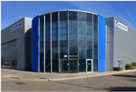
European Headquarters & Production Facility, Southampton, UK
